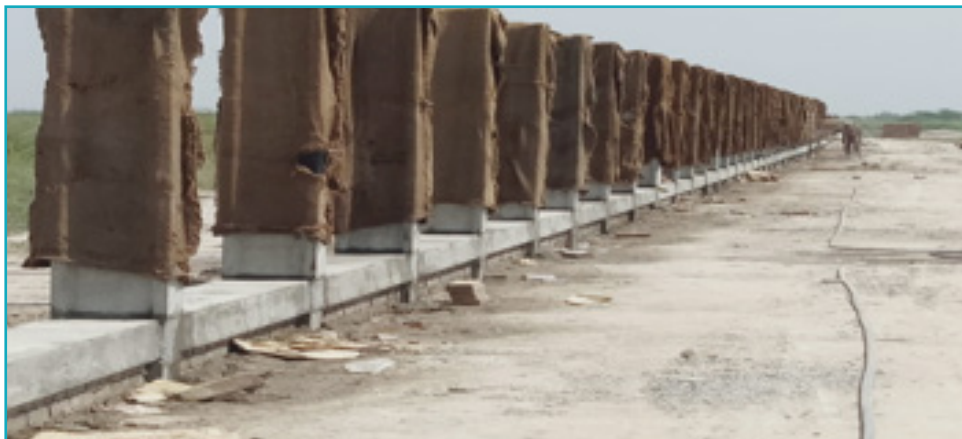
Construction of Boundary Wall Pillars (West Side) at New Campus
