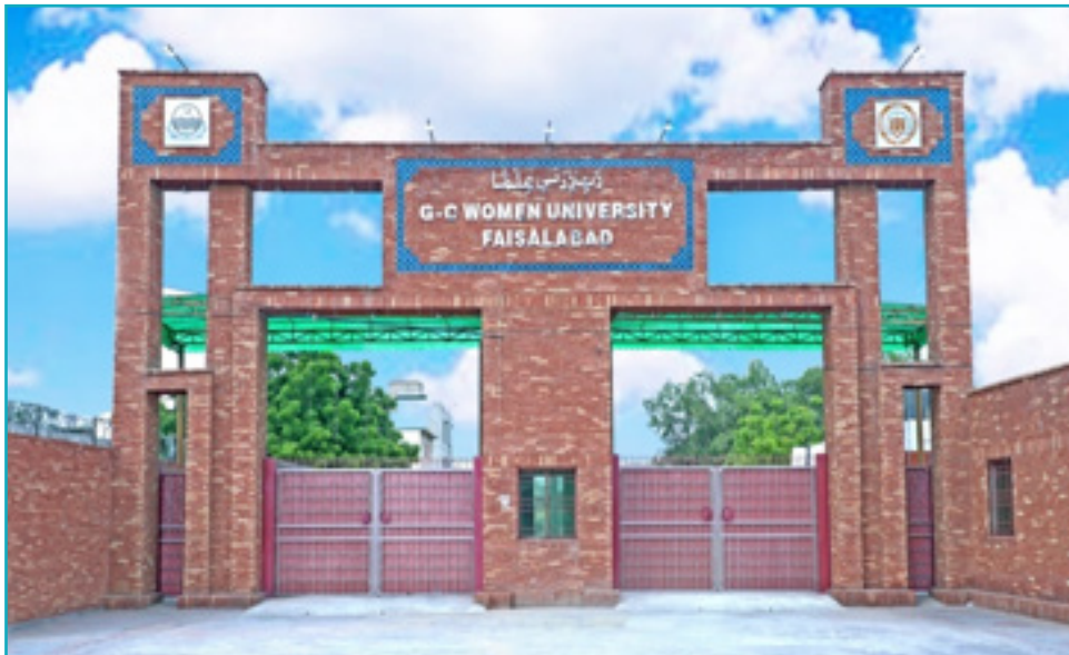
Construction of Main Gate, Electrical Installation and Security Room
